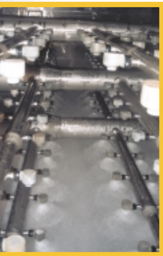
Figure 4: Nozzle arrangement in an SO 2 scrubber
